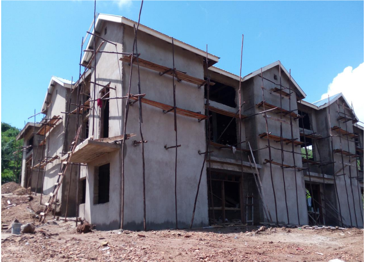
Examination hall in plastering stage
